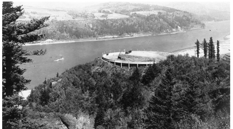
Photo courtesy of the Oregon Dept of Transportation
